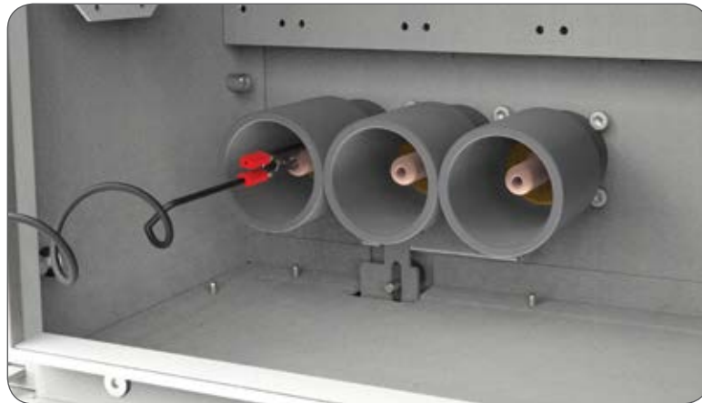
Figure 19: Front view of Cable Testing Compartment
