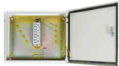
Shrouded Busbar chamber Figure - 9
