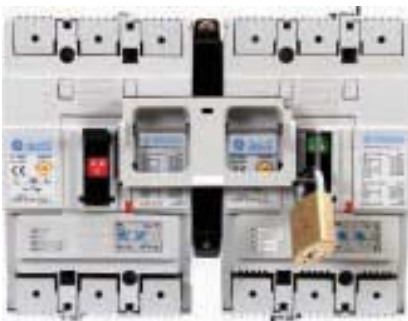
Slide Interlock Installed Between two MCCBs
