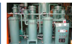
Construction of 380kV Shoiba-3 Substation
