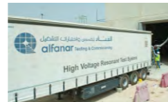
King Abdullah Financial District 132kV Substations (4 Nos)
